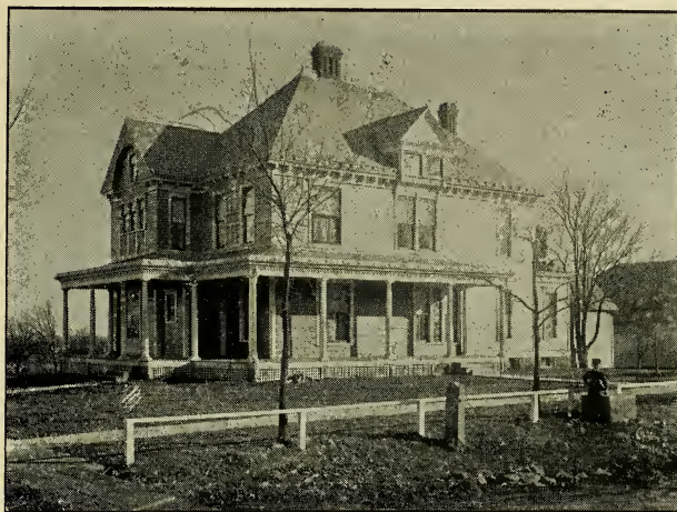
RESIDENCE OF SEWARD GRAHAM.
